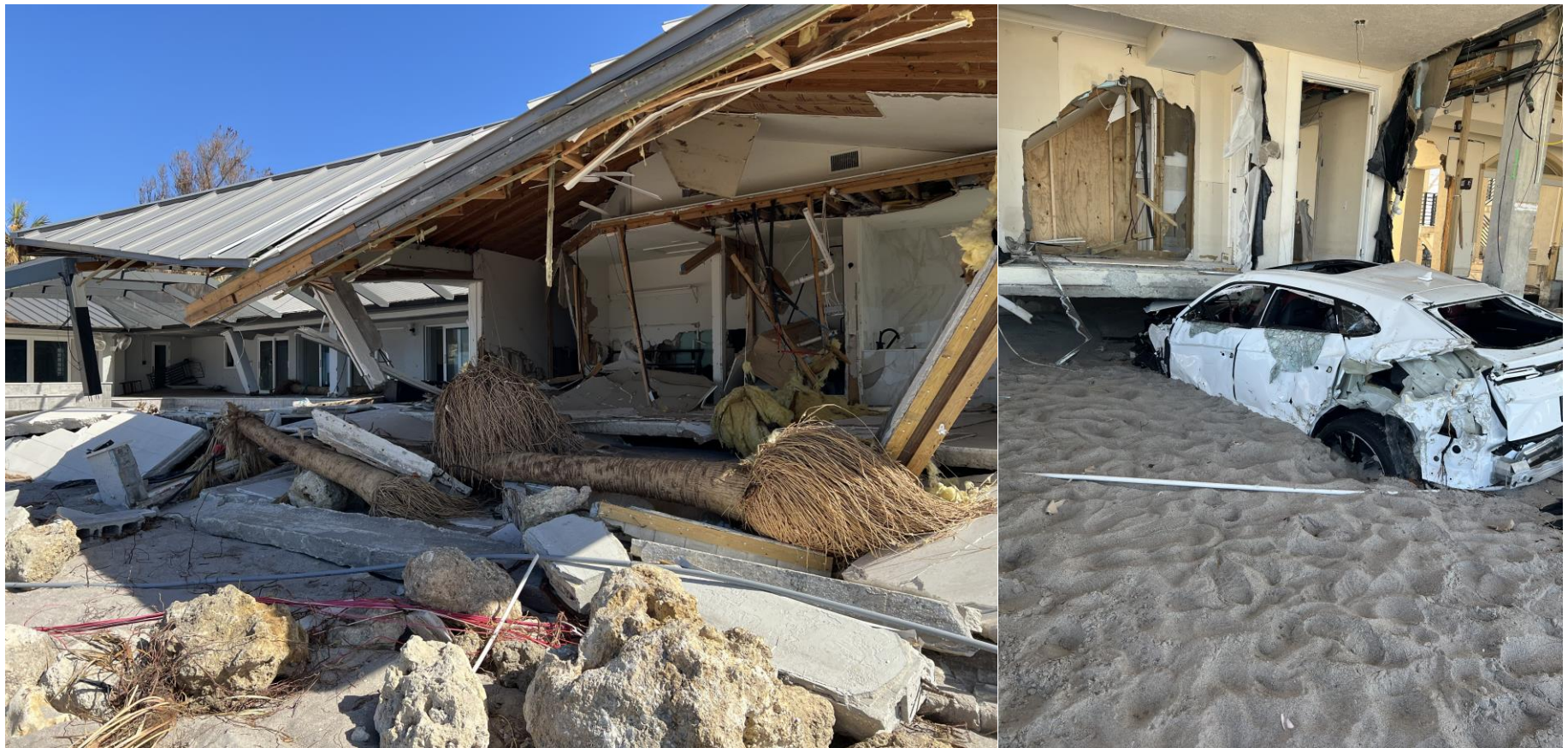
Figure 8. Storm surge damage due to Hurricane Milton on Manasota Key, Florida. Images taken by NWS survey crews on Manasota Key.
