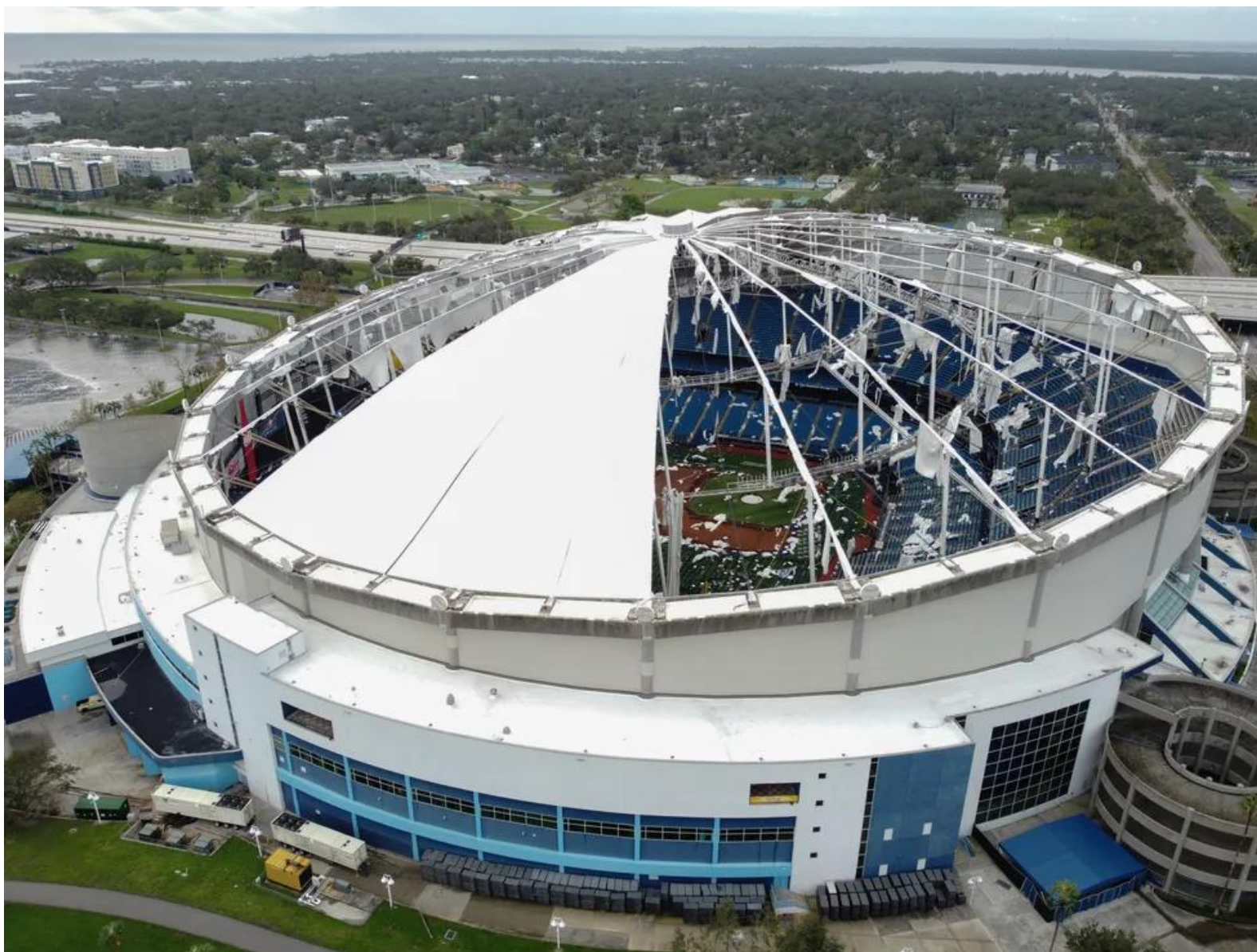
Figure 14. Roof damage to Tropicana Field in St. Petersburg, FL caused by Hurricane Milton. Image courtesy of USA Today, Bryan R. Smith, and Getty Images.
